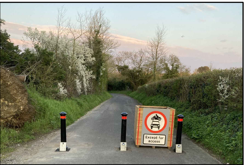
P6 Traffic calming measure - modal filter
