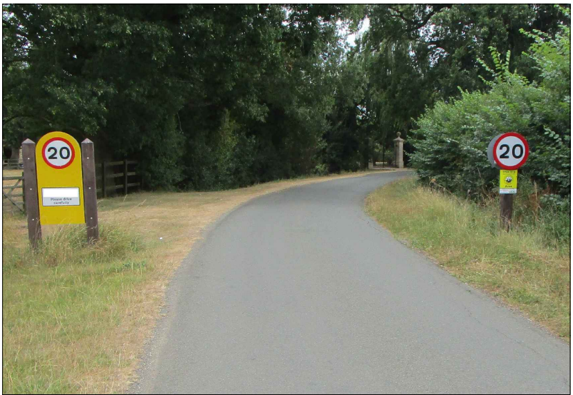
P1 Traffic calming measure - gateway and speed limit sign
